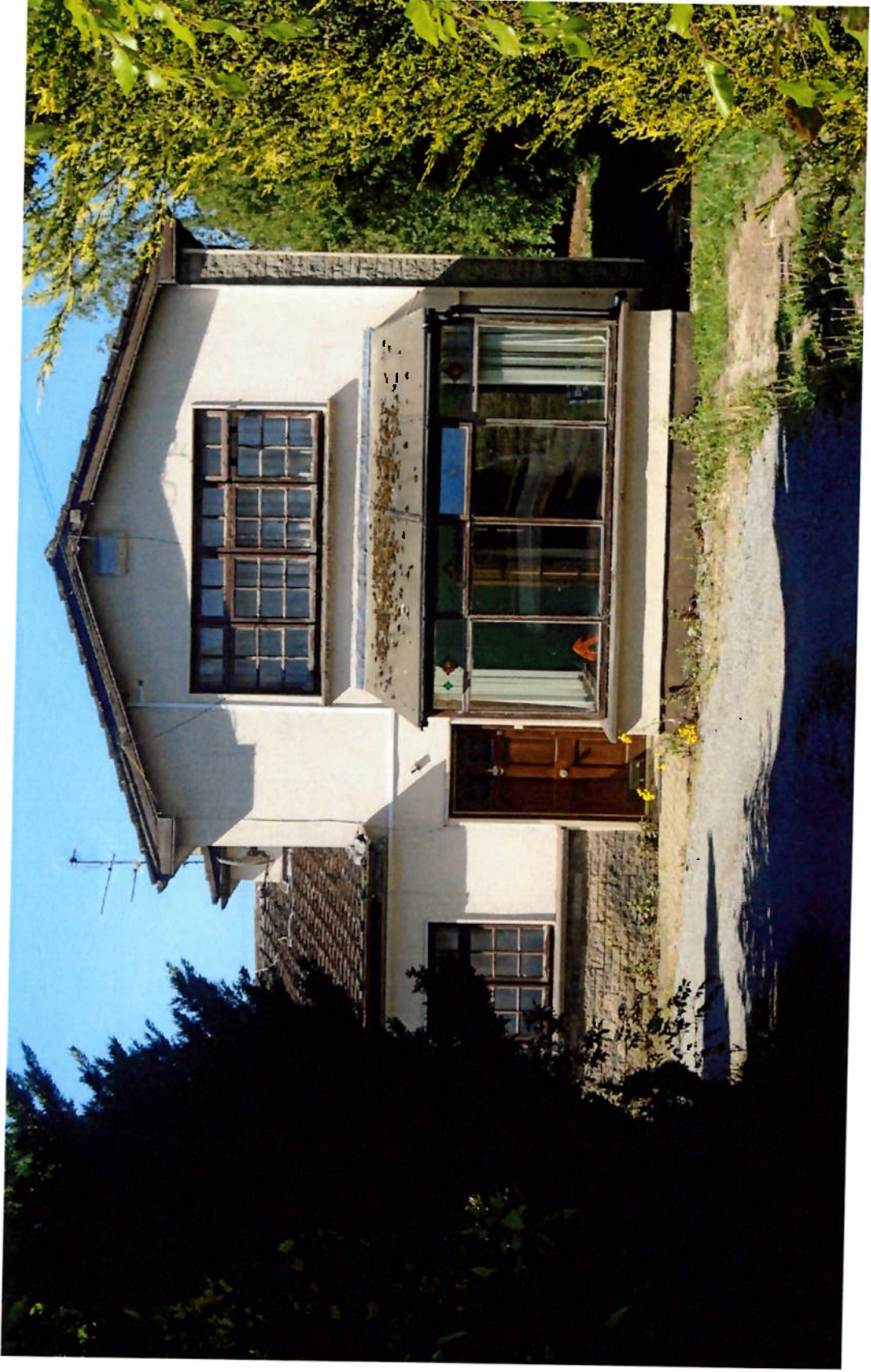
Photo 14: House to be demolished
